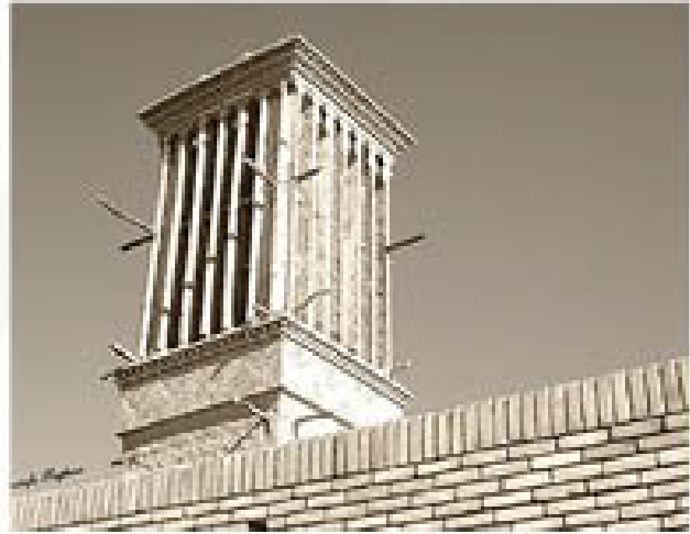
Vertical element- Wind Tower in traditional architecture design as a significant function and design solution
