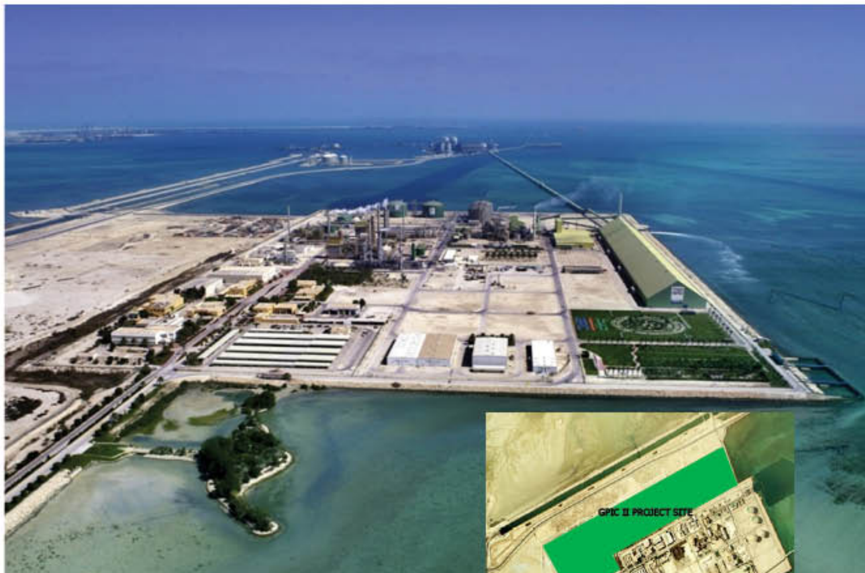
Existing GPIC Site Aerial view
